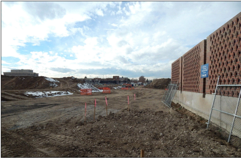
Figure 5: Demolished Site Listed as Provider's Practice Location
